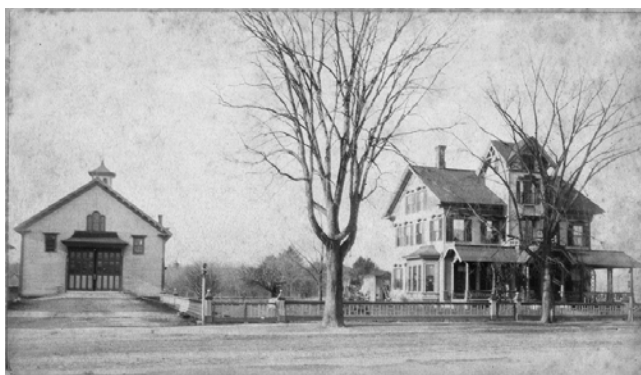
Home of Dewitt C. Remington with barn. Main Street, Harrisville, circa 1900. Courtesy of C. O. Remington III
